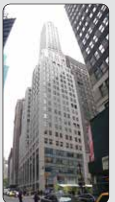
Fujitsu General Solution Centre "THE AIRSTAGE"
