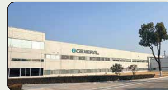
GENERAL Air Conditioning Manufacturing (Thailand) Co., Ltd.
