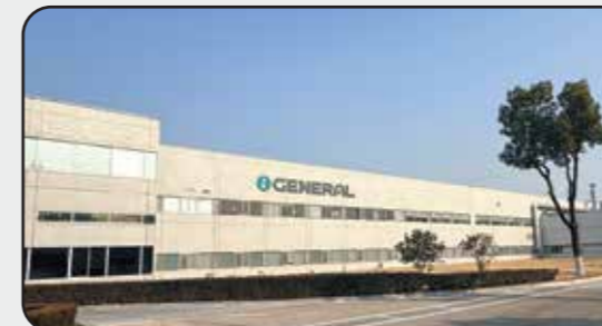
GENERAL Air Conditioning Manufacturing (Thailand) Co., Ltd.
